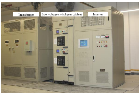
Fig.4 Photo of the PWM regenerative inverter system
